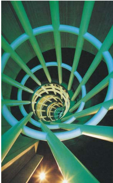
185 | Sendai Mediatheque | View into structural column | Toyo Ito | 2001
