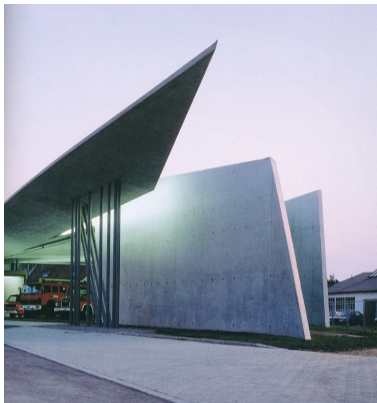
162 | Vitra Fire Station | Exterior view Zaha Hadid | 1990 - 1994
