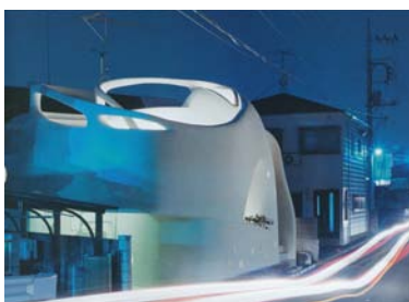
144 | Truss Wall House | Street view Ushida Findlay | 2003
